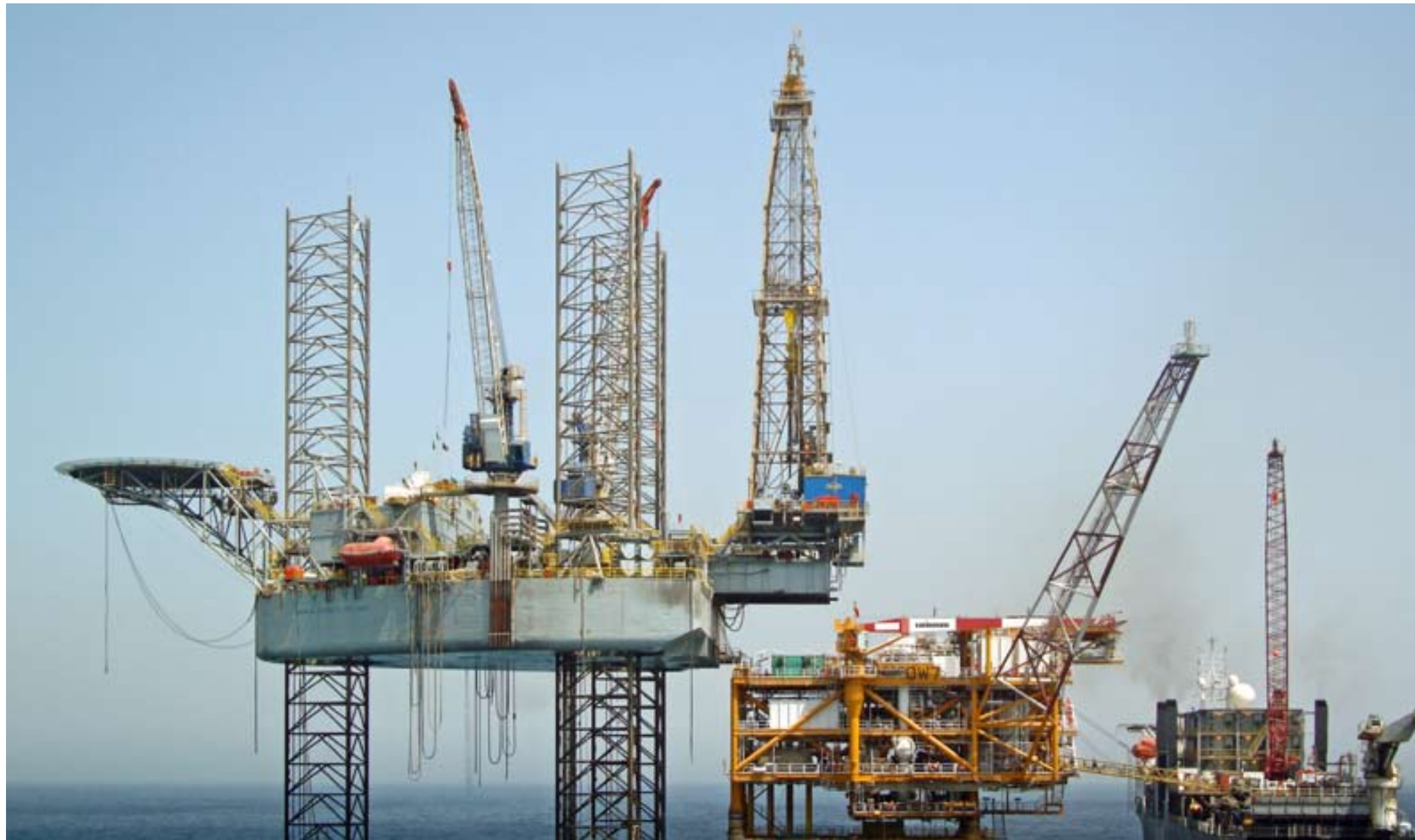
Drilling rig Noble Kenneth Delaney rigged up over WHP-7. M/V Agile, dynamic positioning support vessel on hire to, J. Ray McDermott in position alongside WHP-7.
