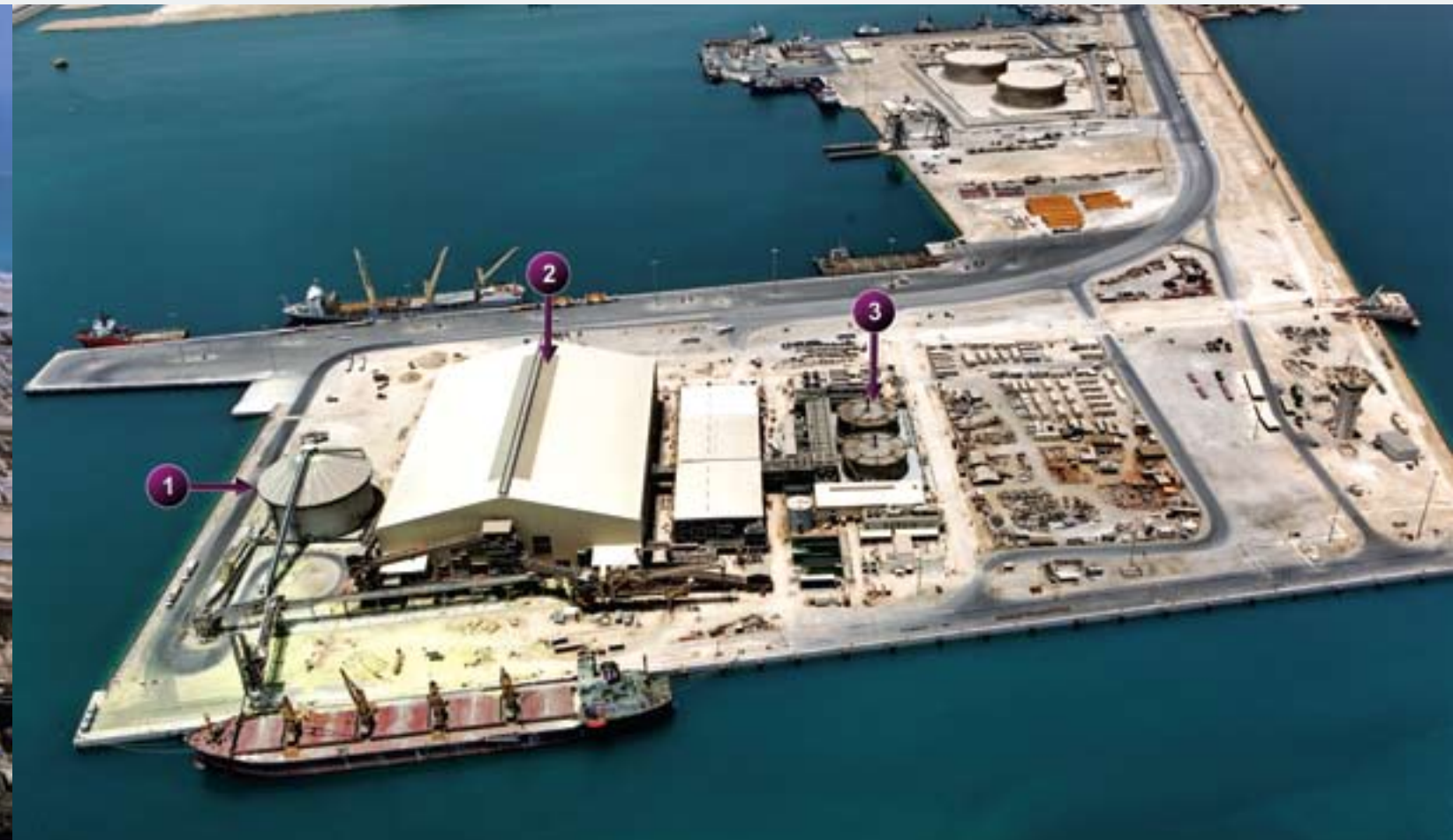
1- Existing Sulfur Silo Storage 2- CSF – Sulfur Storage Building 3- Granulators
