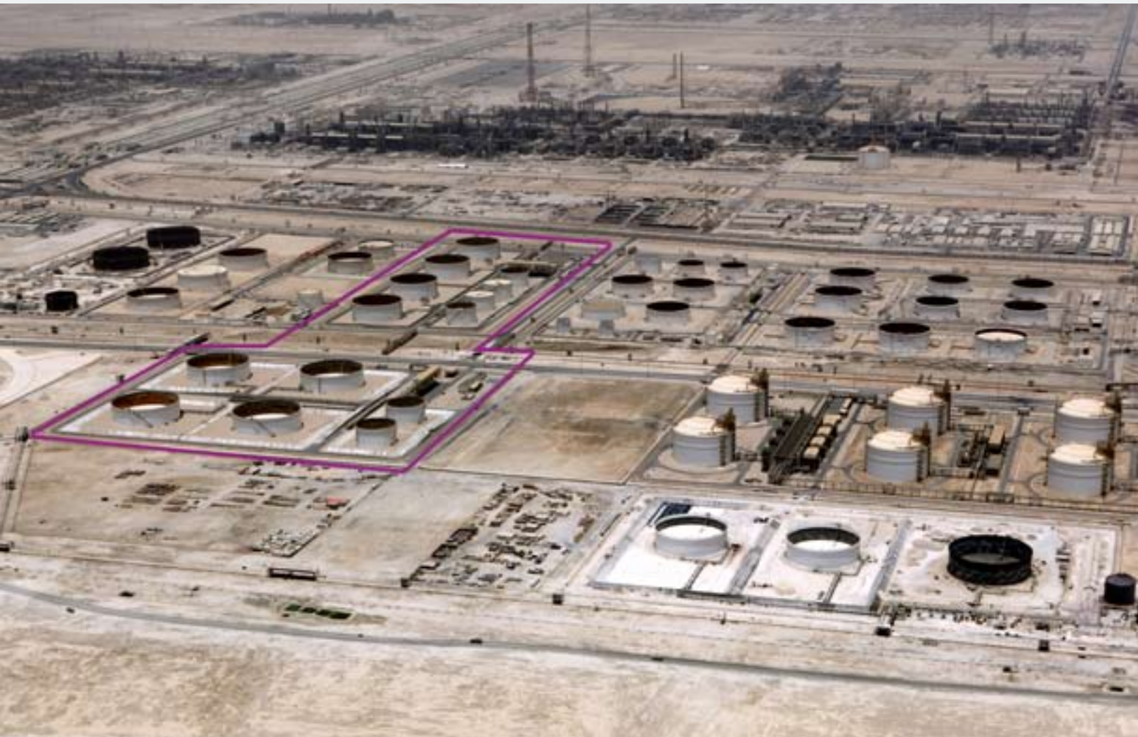
Aerial view of Common Condensate Storage and Loading Facility (CCSL)
